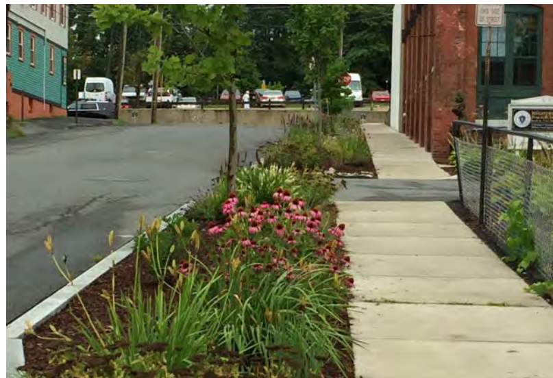
Vegetated swales, like these rain gardens on Olive Street in Greenfield, are one of many solutions to stormwater management discussed in the Town of Greenfield's Low Impact Development: A Developer's Guide.
