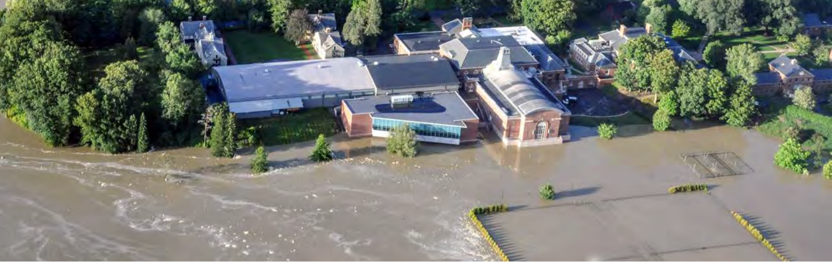
Facilities on the Deerfield Academy's campus were submerged in floodwaters for weeks following Tropical Storm Irene.
