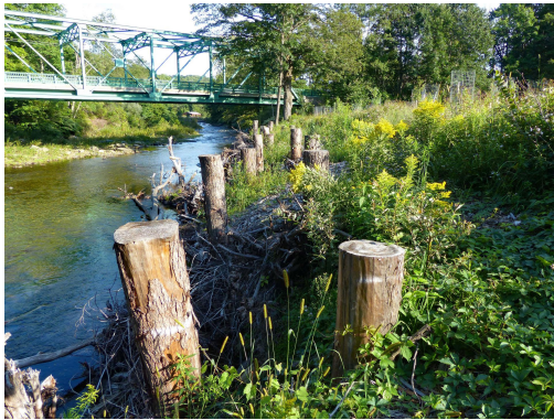
North River Restoration – monitoring photo, one year later
