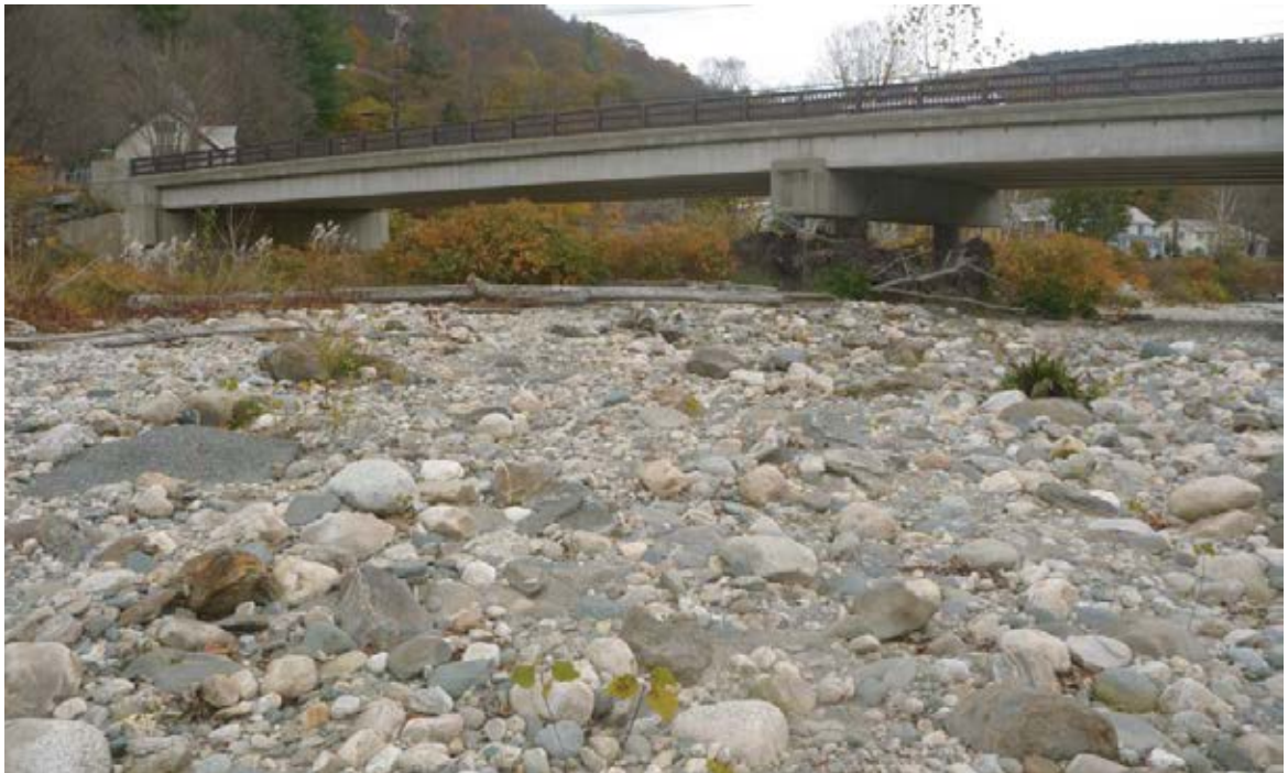
North River Mainstem Sediment Management Project - Photos of a) 50-foot high mass failure opposite the Barnhardt Manufacturing plant on North River Mainstem and b) sediment accumulating around the center pier of the Route 112 bridge.
