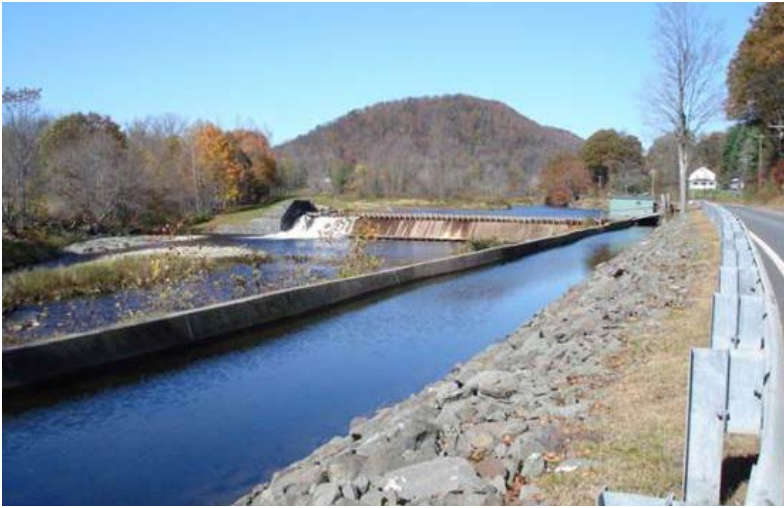
Conditions on the North River, just below the confluence of the river's East and West Branches, prior to Tropical Storm Irene included a dam, canal and armored bank with Rte. 112 in river corridor.
