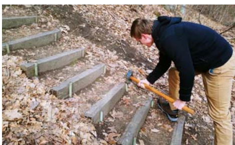
Nate countersinks those annoying rebar.
